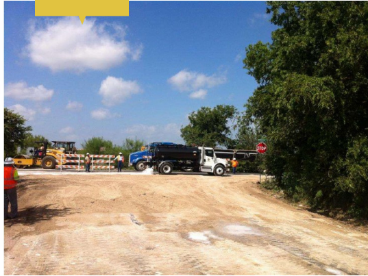
First application of Top-Seal White
