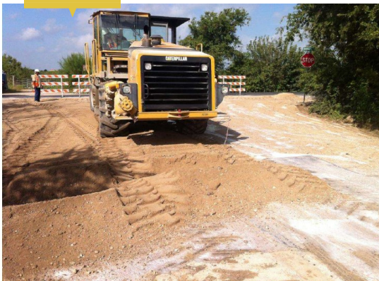
Motor Grader TSW mixing with the soil
