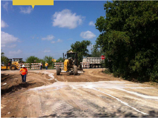
Motor grader after the second application
