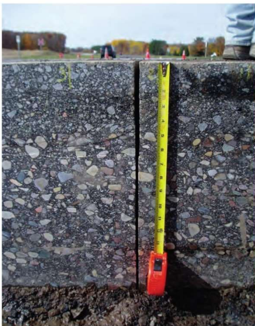
Different Asphalt Mixtures in the Pavement Structure
