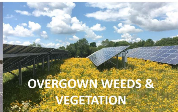
GROUND ALBEDO FOR BI-FACIAL PANELS REFLECTED SUNLIGHT
