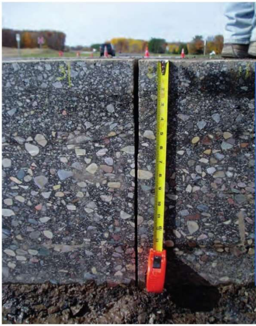
Different Asphalt Mixtures in the Pavement Structure
